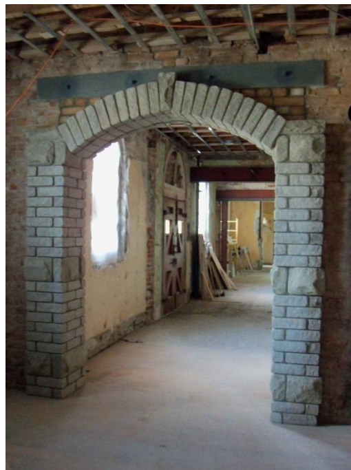
New archway in the main part of the Olde Jail Museum
